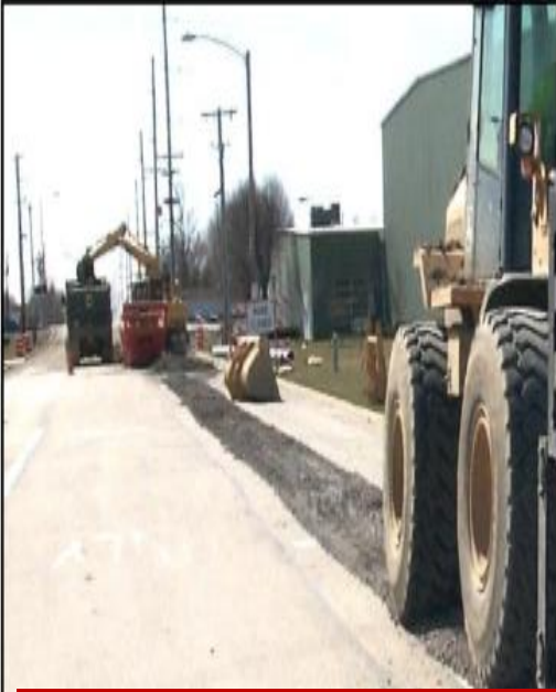
Single pass cut prior to utility line installation
