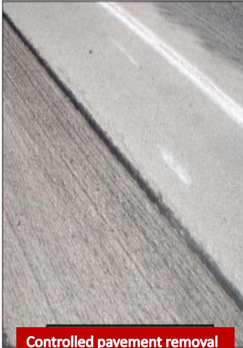
Single pass cut prior to utility line installation
