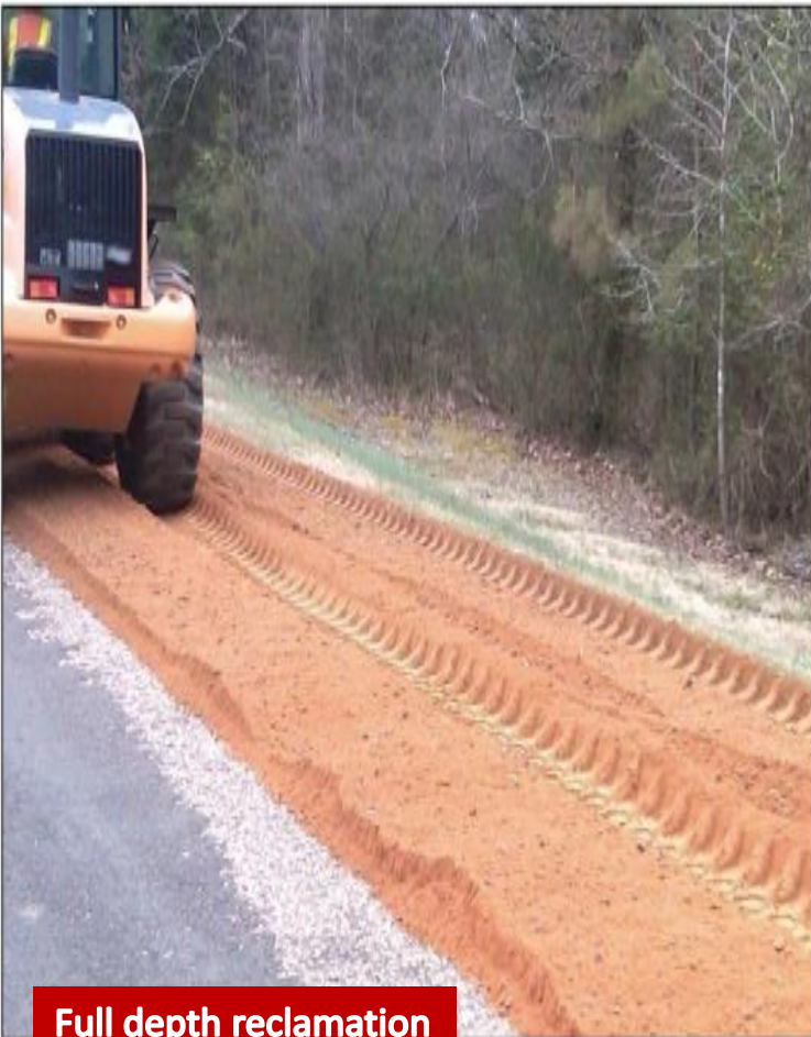
Single pass cut prior to utility line installation
