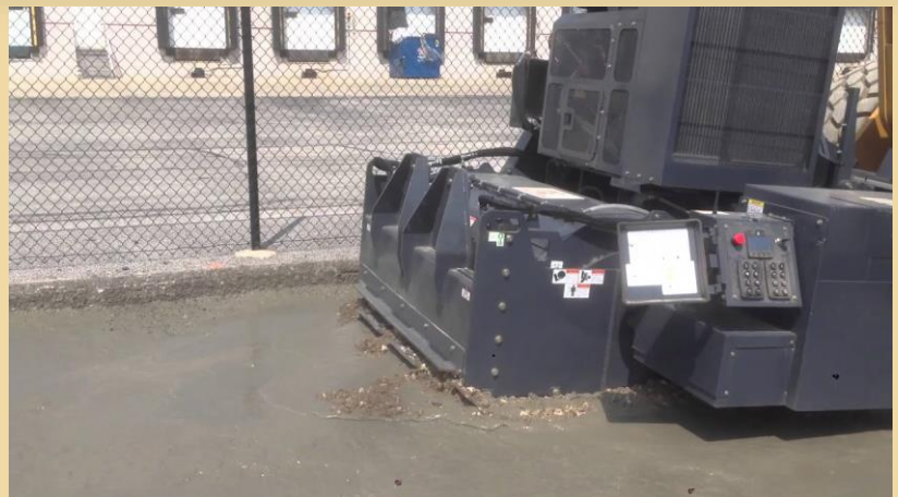
Stabilizing using SLURRY
